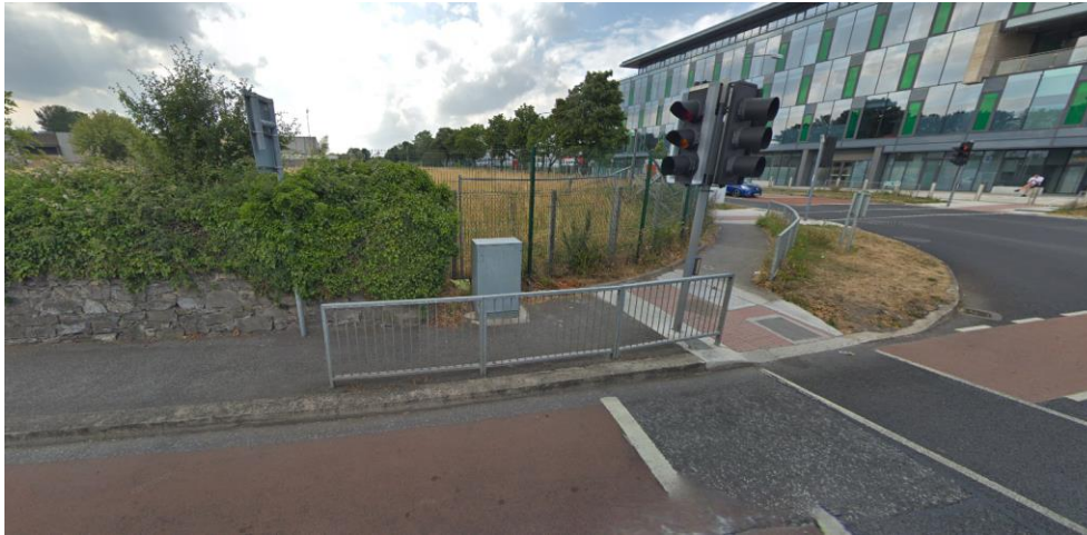
Figure 3.3 – Greenhills Road / Airton Road Junction
