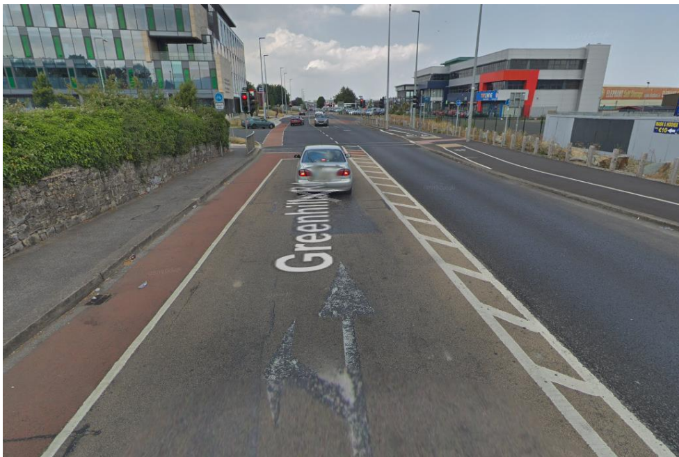
Figure 3.4 – Shared Cycle Lane on Greenhills Road Northbound
