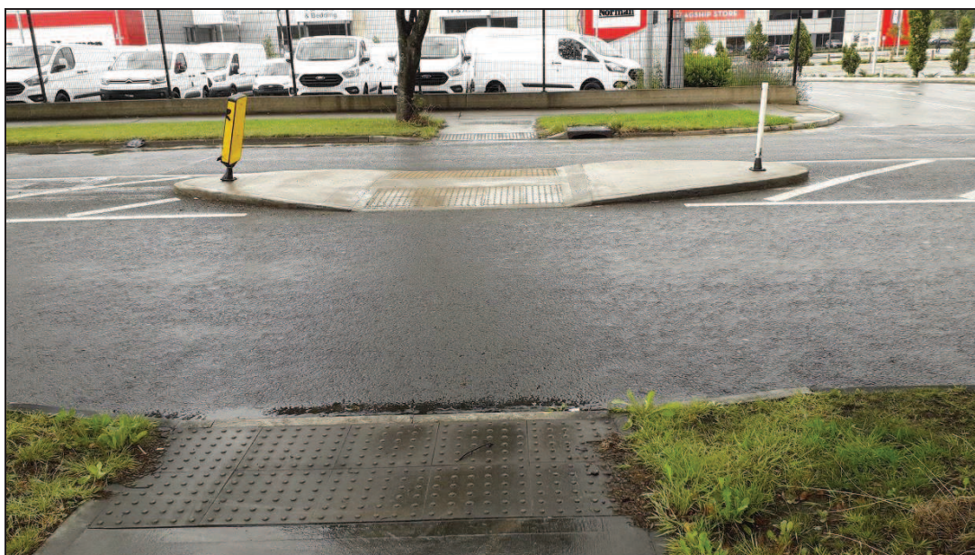
Figure 4.1: Existing Pedestrian Crossing on Airton Road at Location of Proposed Vehicular Access
