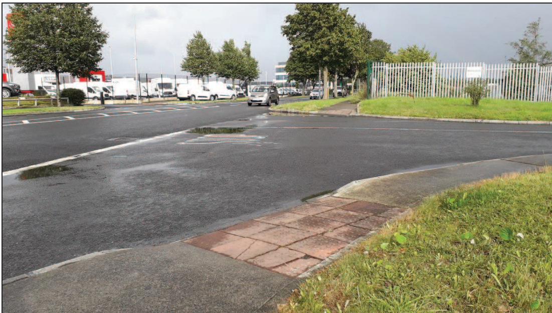
Figure 5.1: Tactile Paving on Opposite Side of Local Access Road off Airton Road to the Immediate West of Subject Site Not Aligned with Proposed Footpath Facilities Fronting the Subject Site on Airton Road
